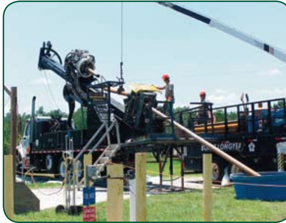
Diagonal Drilling at the F-Area Seepage Basin Savannah River Site
