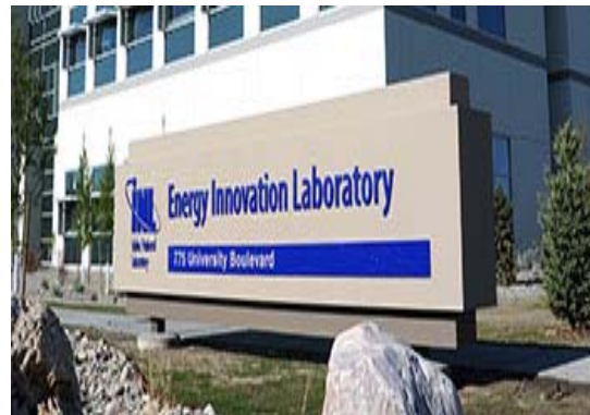
Figure 2. INL Energy Innovation Laboratory.
