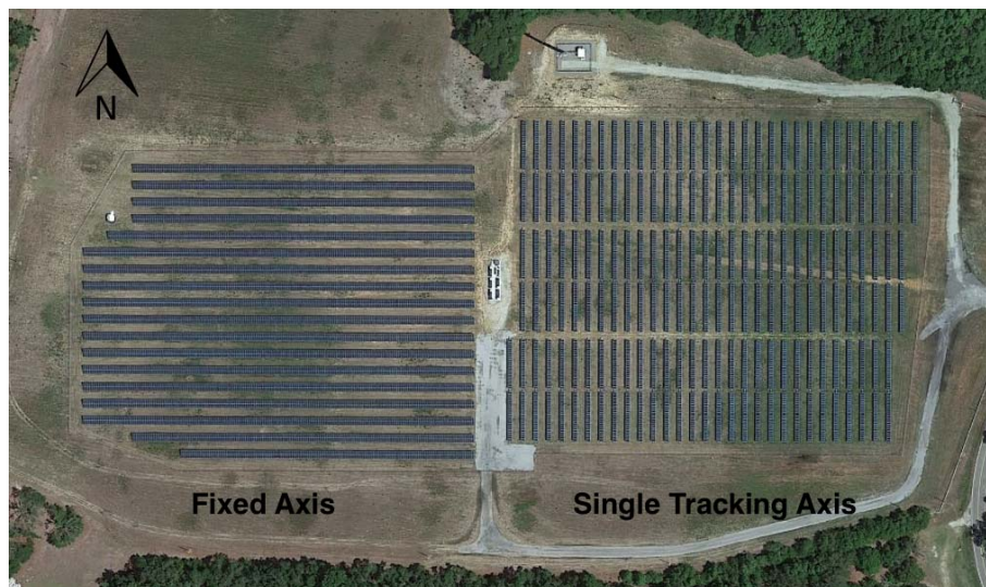
Figure 1. Colleton Solar Farm aerial view.
