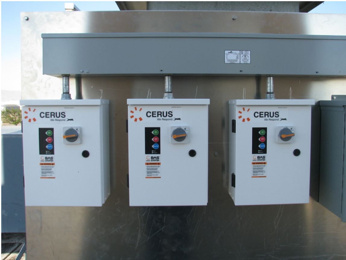
Figure 11. Control enclosures after being assembled.
