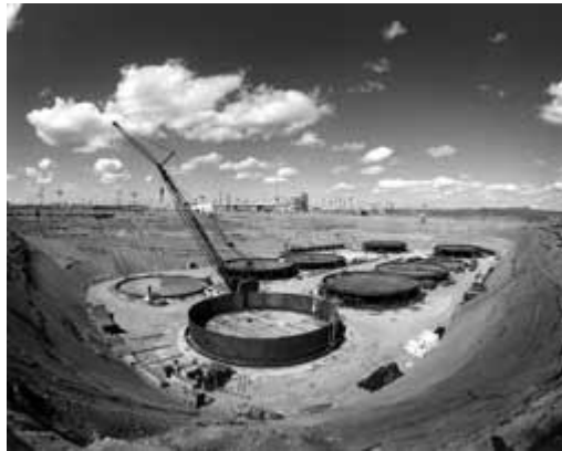
Figure 1. Initial construction of Hanford tanks.
