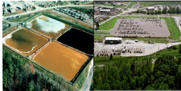
Figure 2. S-3 Ponds site before and after being paved.
