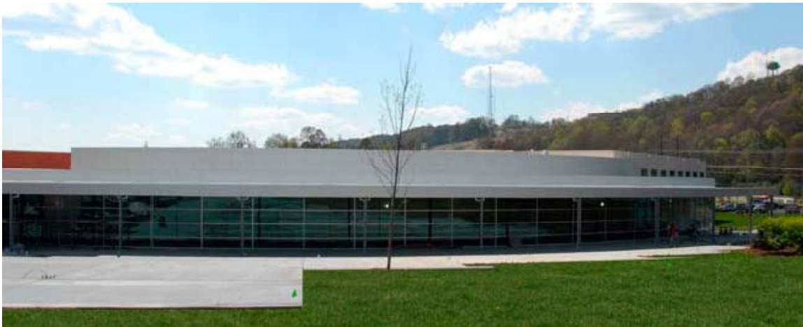
Figure 1. Y-12 New Hope Center, Oak Ridge, Tennessee
