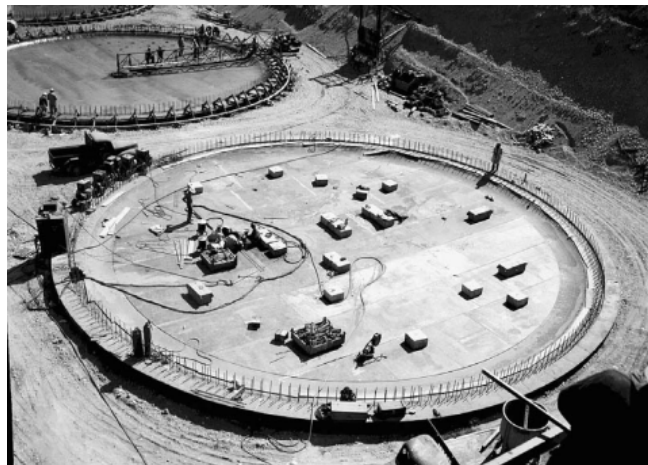
Figure 4. Typical SST basemat during construction of BX tank farm. Taken from [1]
