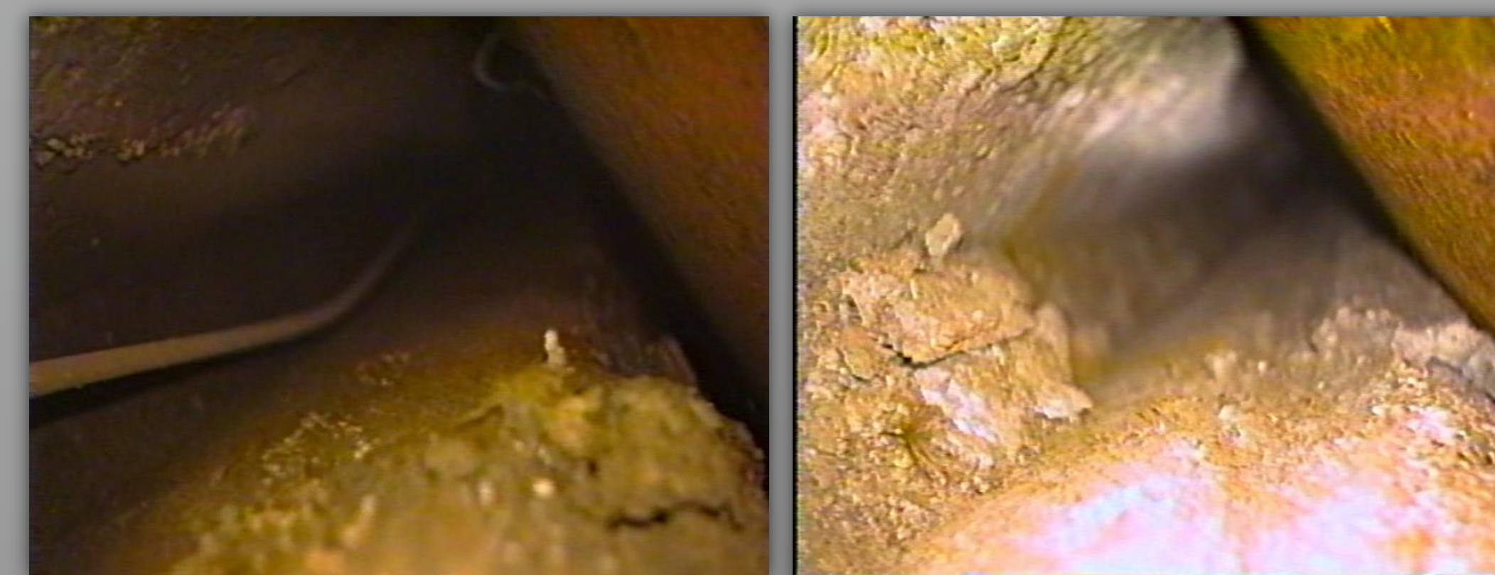
Actual images of cooling channels representing expected conditions
