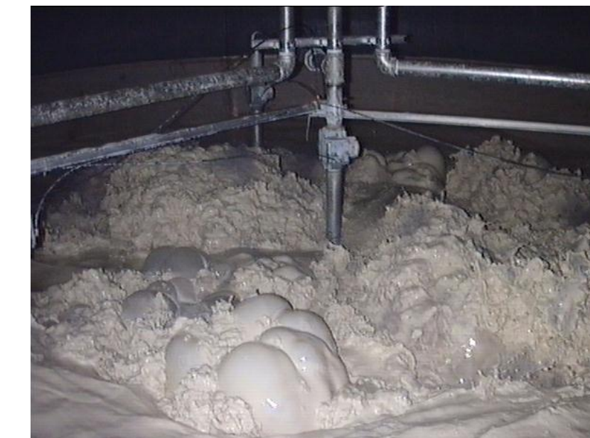
Rising bubbles mix slurry
