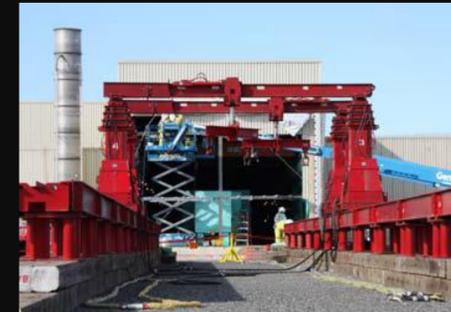
**Challenge:** Physically separating the hot cells weighing 75 and 230 tons from the facility structure and transporting them to the ERDF
