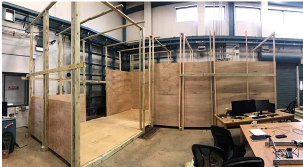
Figure 2. Construction of the section of the CAEX tunnel.
