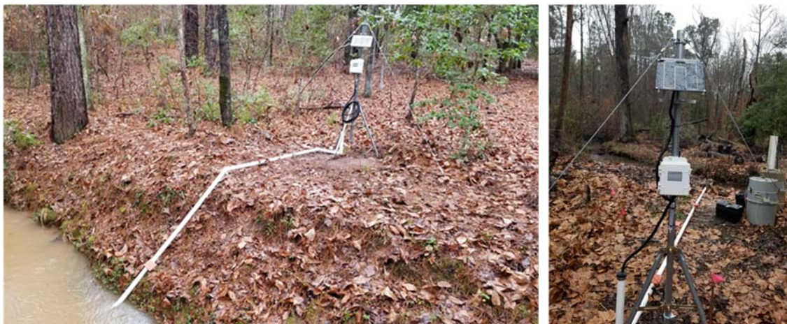
Remote monitoring stations being installed at SRS.
