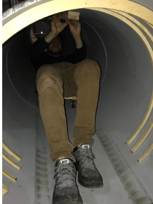
Figure 2. Wooden rings being installed inside the pipes for testing.
