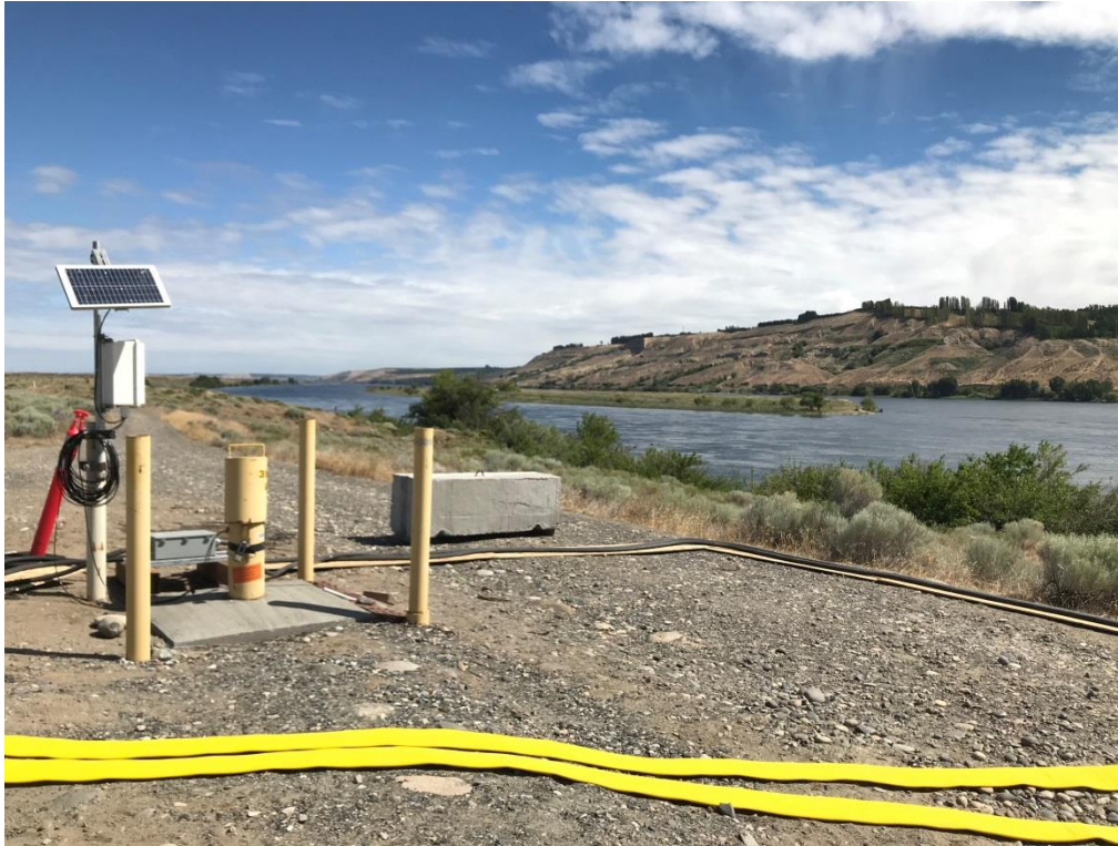
Figure 16. One of the 48 wells (painted yellow) dug into the subsurface of the FF-5 Stage B, 300 Area treatment field (Columbia River pictured at the right).
