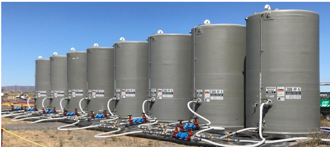
Figure 15. FF-5 Stage B polyphosphate tanks in the 300 Area treatment field.
