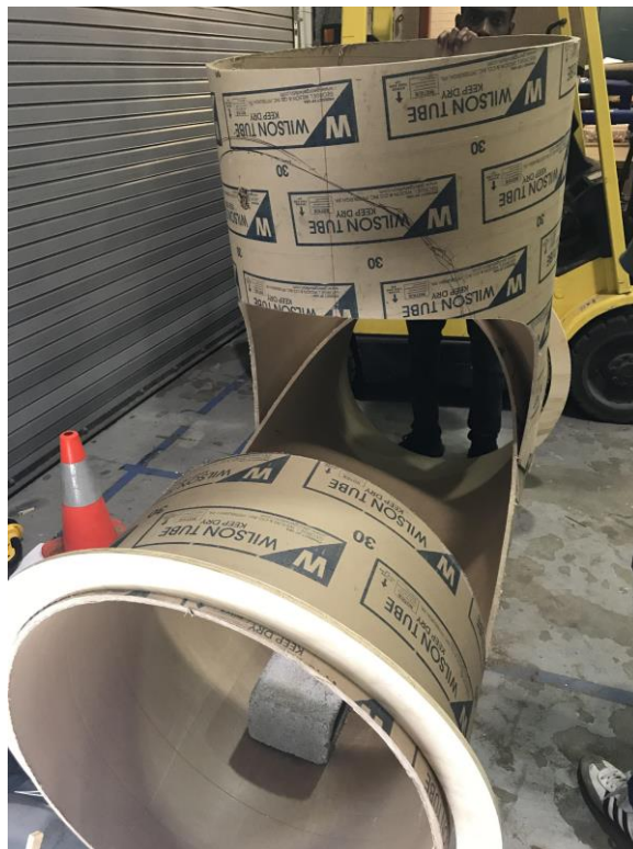
Figure 3. Swept-t pipe section under construction.
