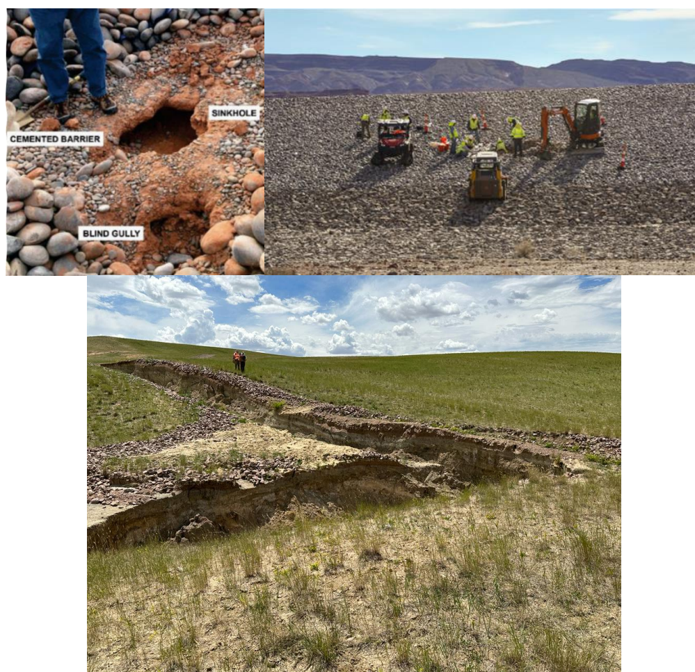
Figure 2. LM disposal cells degradation at Mexican Hat (Top) and Shirley Basin South (bottom).
